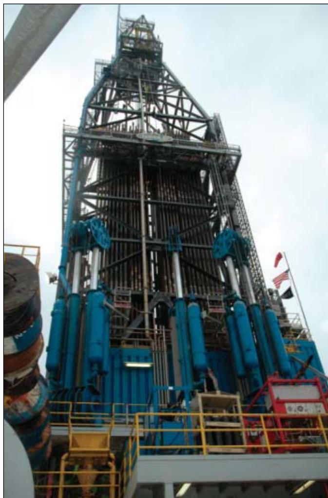
Pipe stands ready in the derrick of Noble Drilling Corp.'s Amos Runner semi-submersible, drilling in Green Canyon Block 955 in December 2006 (photo by Nina M. Rach).
