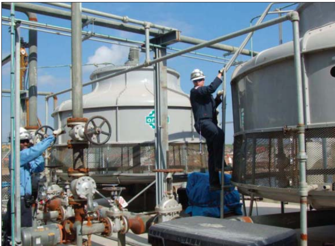
Workers commissioning cooling towers in the Galveston Bay Biodiesel LP plant in Galveston, Tex. The plant is in production. Chevron Technology Ventures is an investor in the plant run by Bio Select Fuels LLC. Photo from Standard Renewable Energy LLC.
