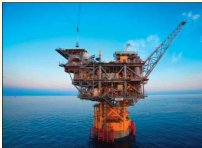
TLP installed at Neptune field
