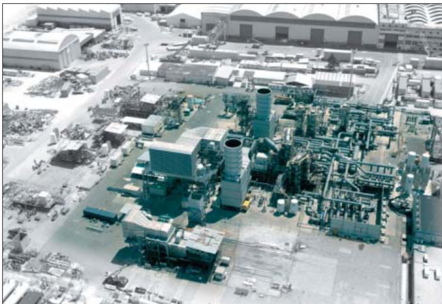
Before shipment, each of the three compressor strings underwent a full power string test at Massa. These tests sought to replicate plant site configuration (Fig. 8; photograph from GE Oil & Gas, Florence).
